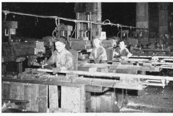
7) Alpha brass and other alloys not readily worked hot and which are to be made into rods or wire are cast in pointed beanpole shapes. These go through the same processes that the bars follow. They are overhauled much the same way. Here Giuseppe Antonelli, Antonio Donofrio and Orfeo Canuzzi attend the Rod Overhauling machines.
